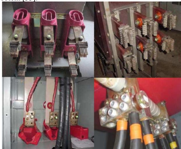
Fig. 8. Wireless sensors installed on finger clusters and cable connections in MV and LV switchgear.
